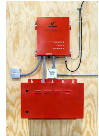
Battery Backup Unit (BBU) and Alarm Annunciator
