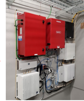
Optical Remote Units (Active DAS)
